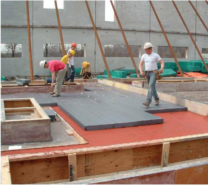
*Four inches of rigid insulation was incorporated into the Tilt-Up sandwich panel wall design. The panels, which were cast on site, used Dayton Superior's P24 Delta Ties to connect the fascia and structural sections through the insulation.*
